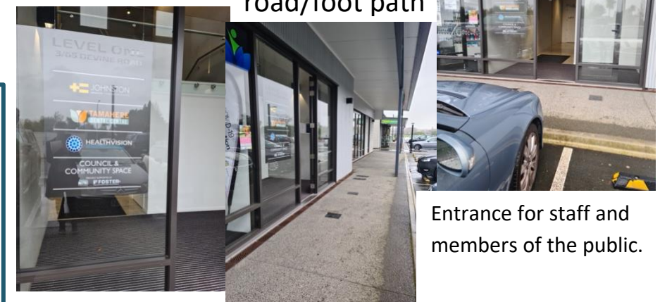
View from the road/foot path
